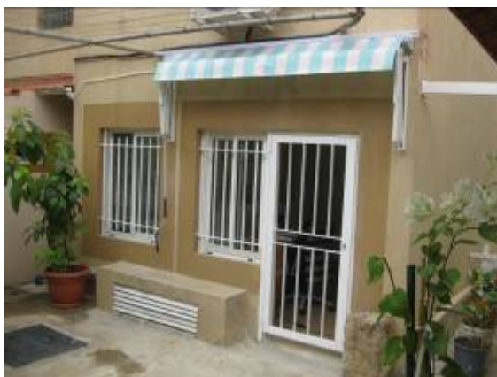
Renovation and aluminum works at the offices, supported by AMT-NL
